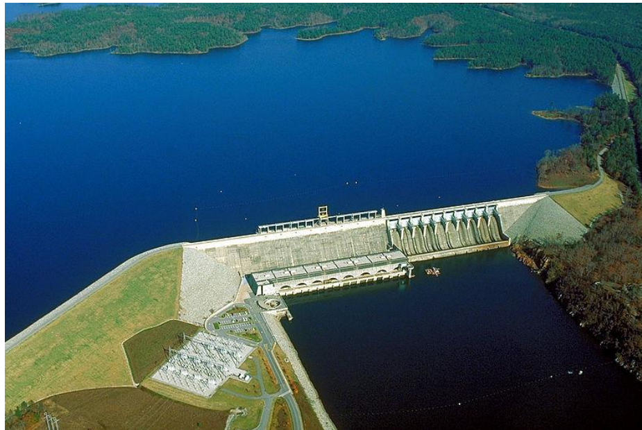
Richard B. Russell (USACE) 300 mW conventional capacity 300 mW pumped-storage capacity (integral)
