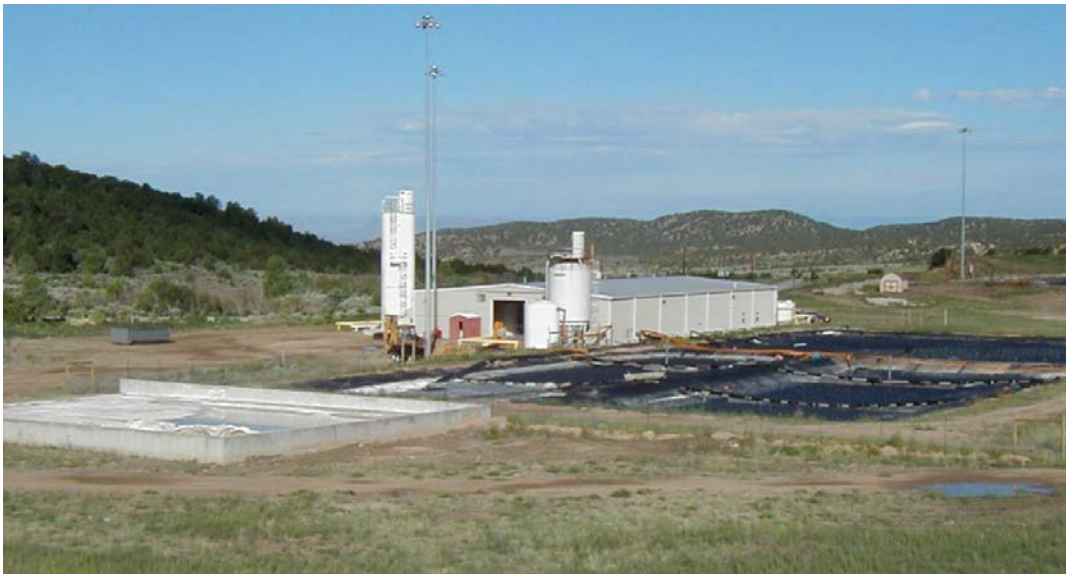
Figure 6 – Rito Seco Water Treatment Facility
