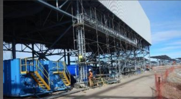
Installing cable trays on the ACC
