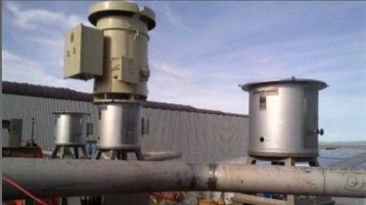
Hot salt pumps erection
