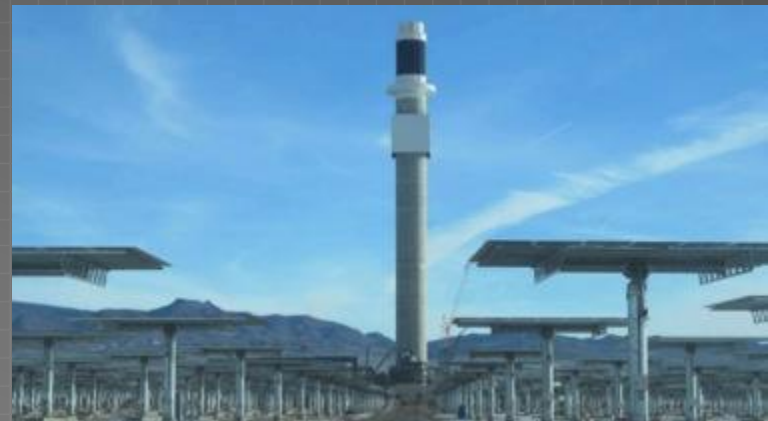
Tower and receiver assembly
