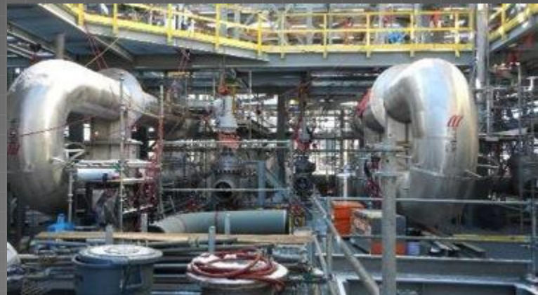
Installing reheat valves
